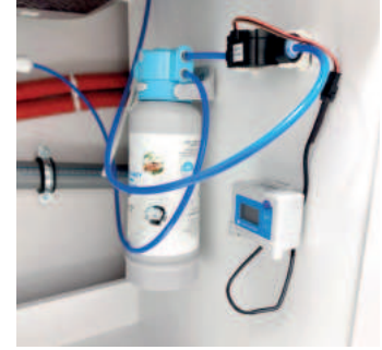
Meter installation example
